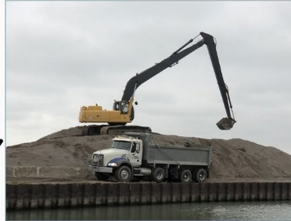
Land-based mechanical dredging at Wheatley
